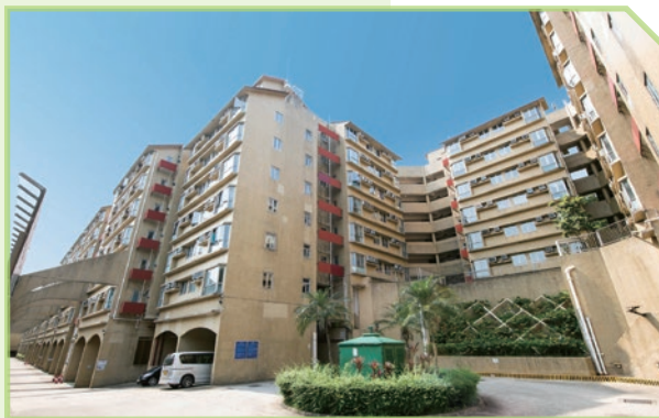
▲ Trackside Villas 策誠軒
